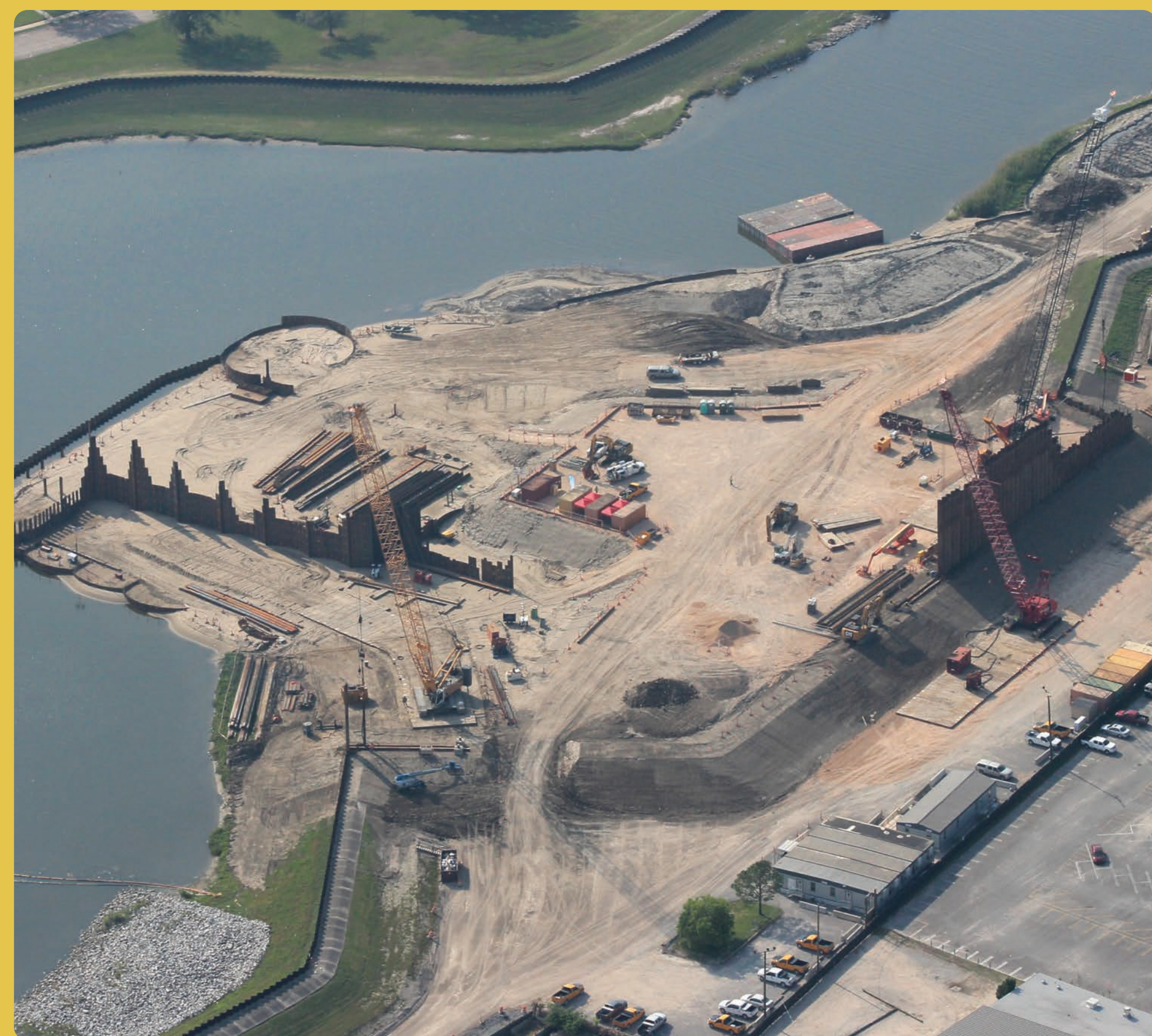
Construction Activity at PCCP
