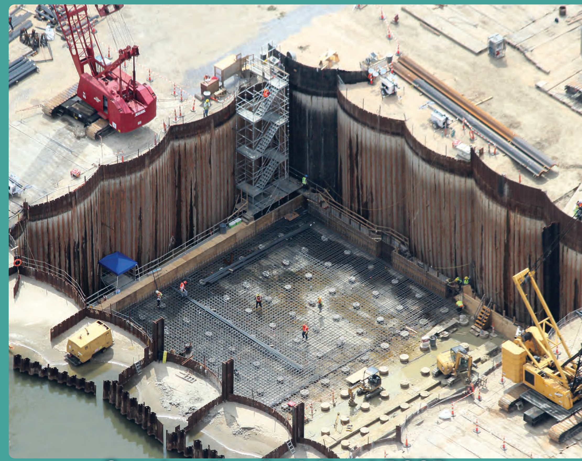
Construction Activity at PCCP
